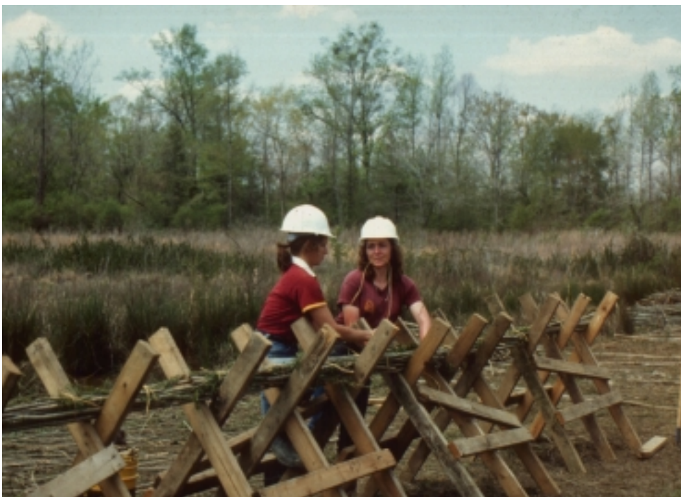
Figure 18-7 Fabrication of a live fascine bundle (Robbin B. Sotir & Associates photo)
