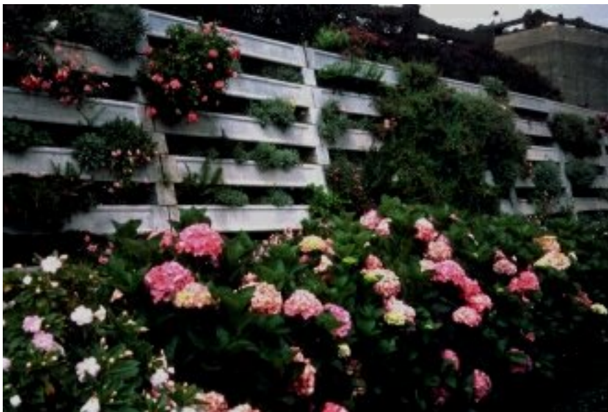
Figure 18-28b Open-front concrete cribwall with plantings in openings
